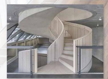
Spiral staircase at the centre of an administrative building of SSB. A filigree wooden staircase has been built around a load-carrying concrete structure.
